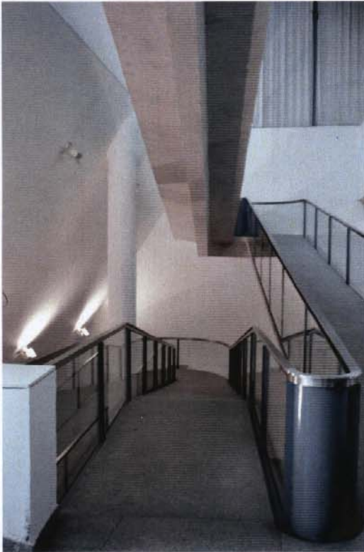
Figure 11: View of the Exhibition Pavilion ramp.
