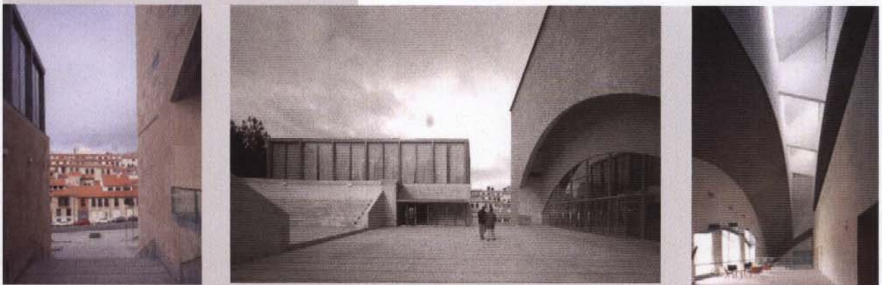
Figure 4 : Building for the conference and exhibition Hall in Salamanca
