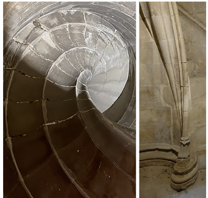
Figure 11. Left. Intrados surface of the Gothic spiral staircase in the Cathedral of Jaen. Right. Central molding (Image by the authors).
