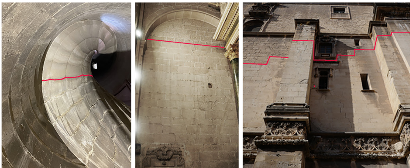
Figure 4. Cathedral of Jaen. Left. Gothic spiral staircase. Center. Wall at San Fernando Chapel. Right. Chevet wall on the east façade. Marked in red is the course of separation between the two construction stages (Image by the authors).
