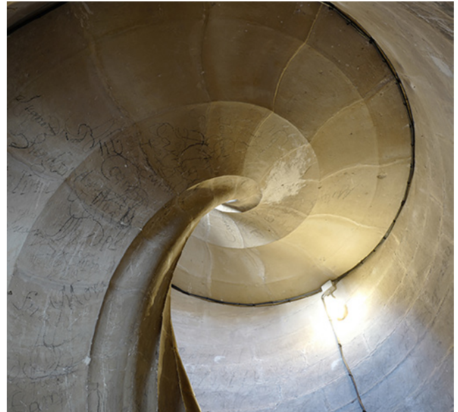
Figure 3. Cathedral of Jaen. Tower spiral staircase. Intrados surface (Image by the authors).
