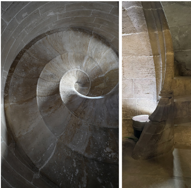
Figure 10. Left. Intrados surface of the spiral staircase in Lonja de la Seda . Valencia. Right. Central molding (Image by the authors).
