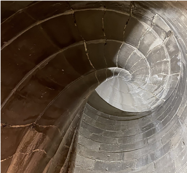
Figure 2. Cathedral of Jaen. Gothic spiral staircase. Left: Intrados surface (Image by the authors).
