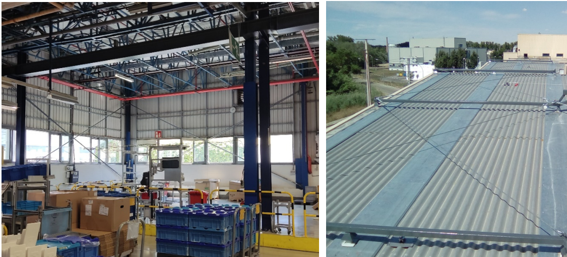
Fig. 3: New bracing system in an existing industrial building
