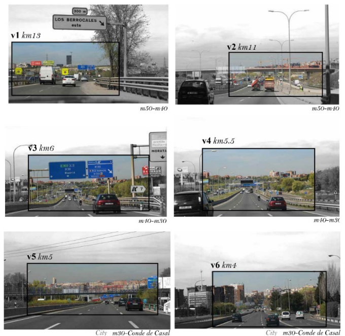
Figure 7: Selection of frames throughout the studied section of the A3 main access road.
