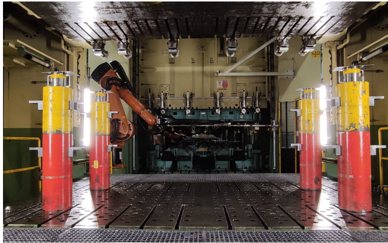
Fig. 6: Test measurement tools installation
