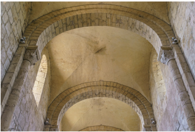
Figure 5. Photograph of a groin vault over the nave of Sainte-Trinité (M. Pfister).
