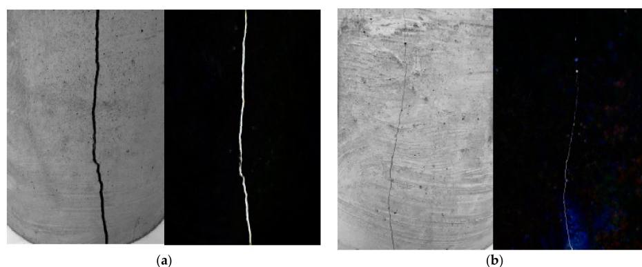
Figure 12. Shrinkage Crack Width (a) Without Fibers and (b) With Fibers [87].
