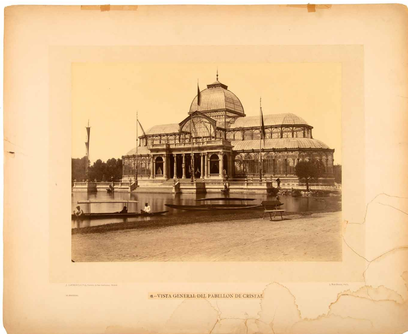
Figure 52: General view of the Glass Pavilion of the Philippine Islands General Exhibition (1887). Author: Laurent y Cía. MNA Collection: FD2857. Photograph taken from the original, photographer: Javier Rodríguez Barrera.
