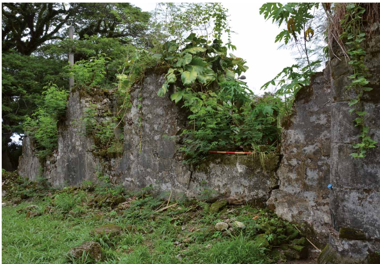
Figure 34: San Dionisio's walls at present. Photo: Sandra Montón for ABERIGUA project.
